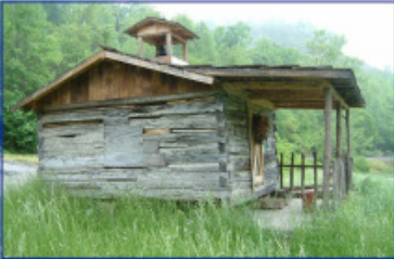
Log building with cupola and bell
